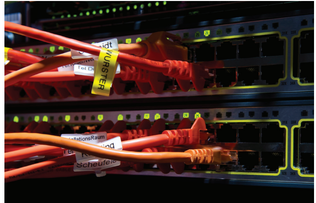
Special formats and materials for cable identification: vertical and horizontal flag, self-lamination wrap around and Heat Shrink Tubes
